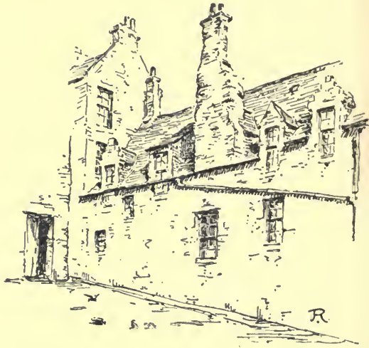
Back of Mackenzie's House, looking into Cant's House.
